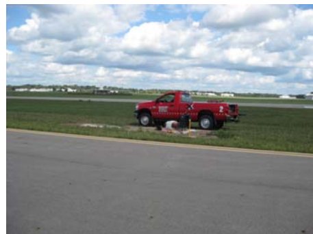
Josh Clamon on airfield installing new Runway directional signage
