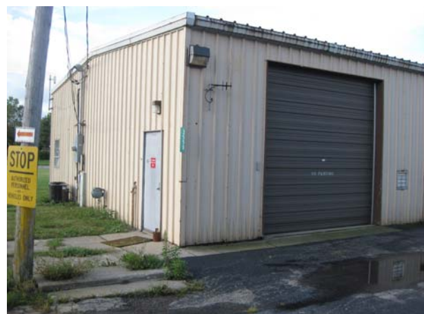
East side of Trybe Building where Jackson Community Ambulance will be housed and construction will take place
