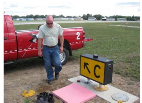
Josh, Airport Technician, working on installing more directional signs
