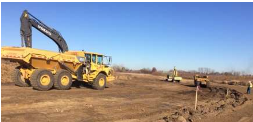
Nearly half way at 90,000 tons removed.
