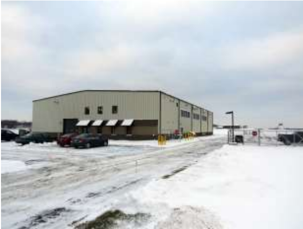
View from Airport Road looking West
