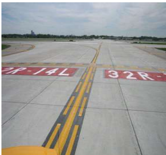
Standard “Hold Short” Runway Markings
