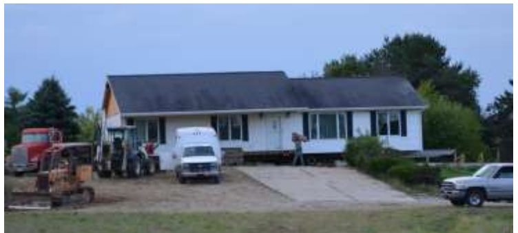
Extensive pre-move preparations.
