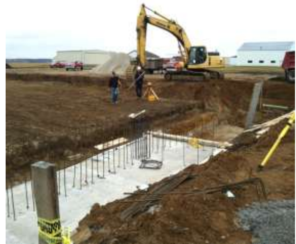
Footing for the SRE building.
