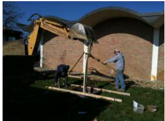
Installing mounting pole in front of the terminal building.
