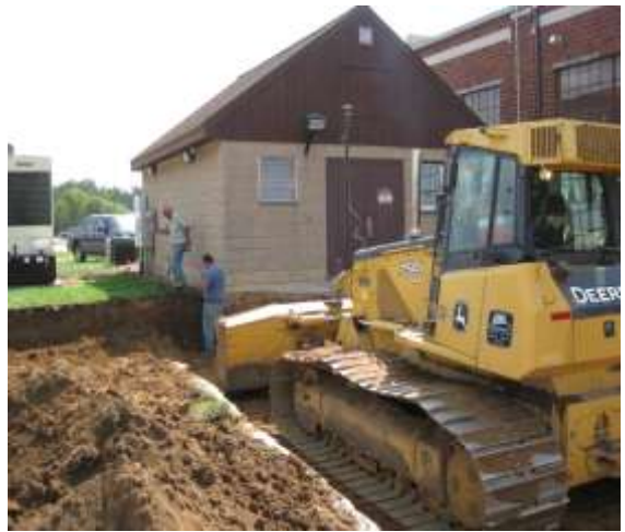
Construction near the airfield electrical
