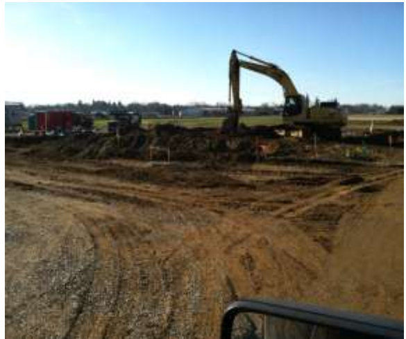
Excavating for SRE footings.
