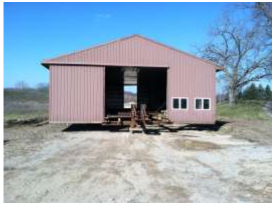
Barn moving made the newspaper too.
