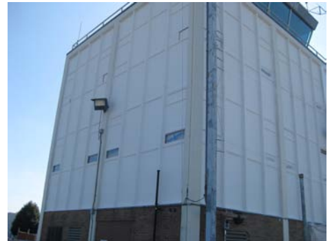
Ceramic Coating on JXN Air Traffic Control Tower
